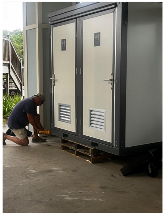
Portable Restrooms Installation
